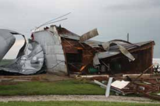
◀ Tornado damage near Harlan in Nishnabotna Valley REC's service territory.
